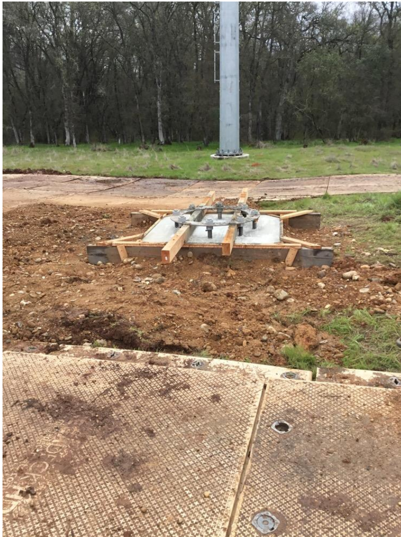
Photo 1: New foundation installed during the reporting period at site 1/11.
