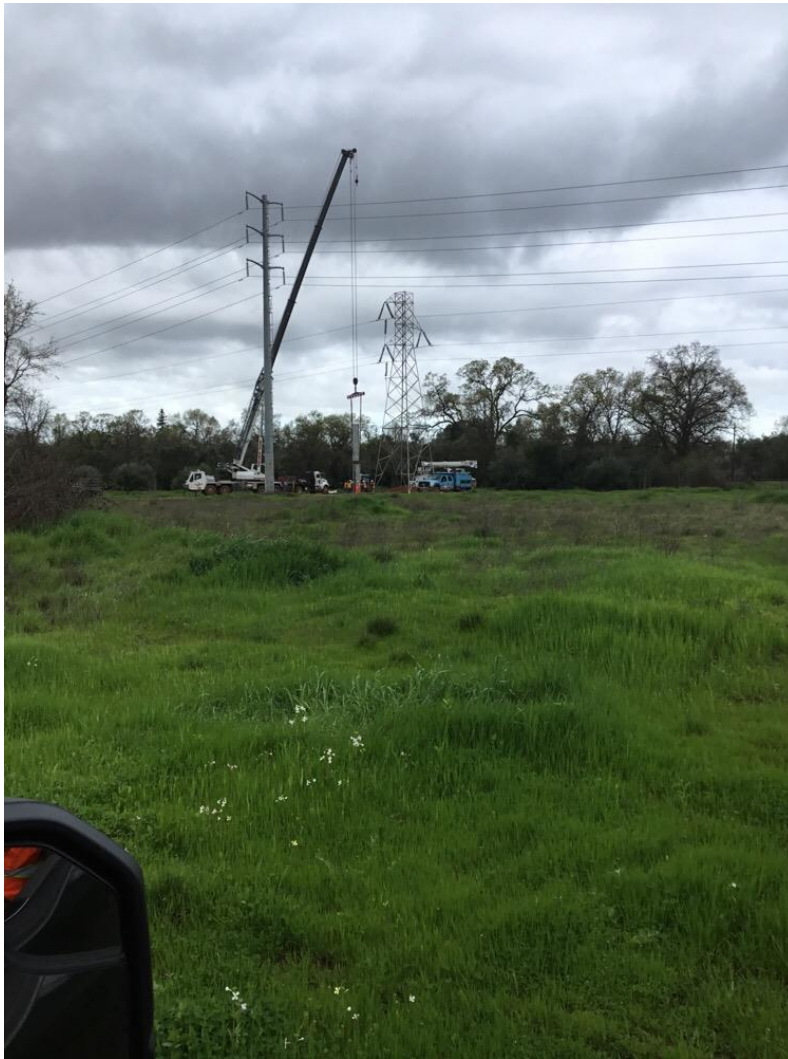
Photo 2: Crews were observed installing a pole base at site 3/28.
